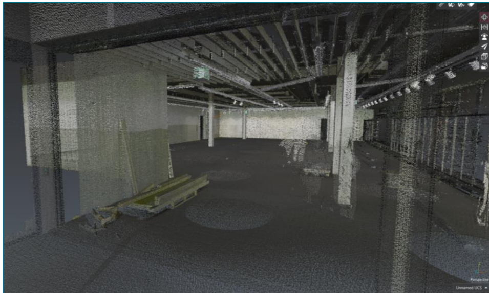
Construction site capture with RTC360 (shopping center)
